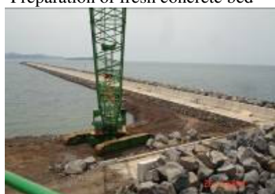
Crown-wall in position
