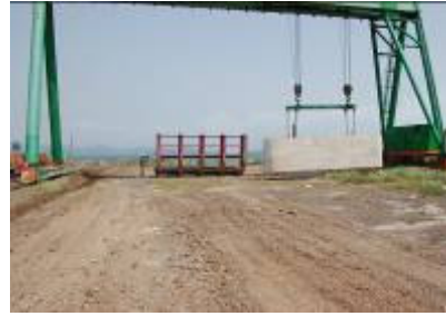
Elements lifted with 60T gantry crane on to turning frame
