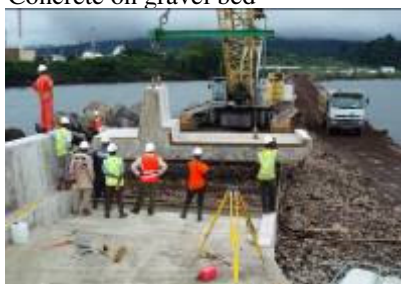
Positioning of crown-wall
