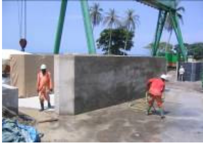
Elements at pre-cast yard with retarder at underside of slab
