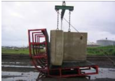
Element on turning frame
