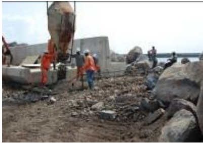
Concrete on gravel bed
