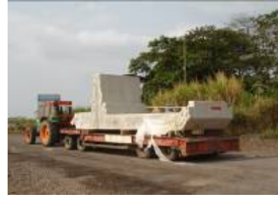
Transport of element to site
