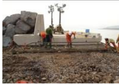
Preparation of fresh concrete bed
