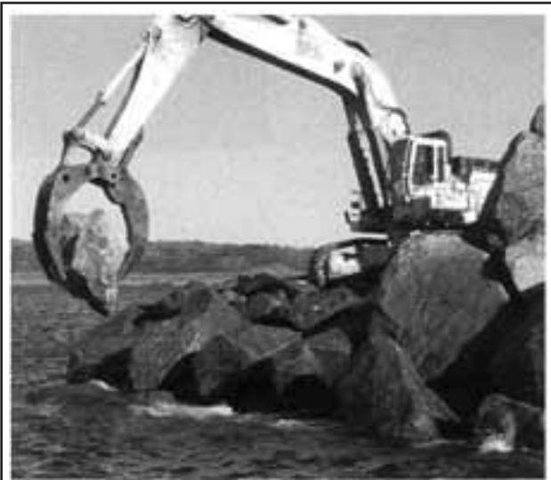
*Figure 11.1. Construction of the Sirevåg berm breakwater, Norway, 2000 – 2001. The 110 ton excavator is placing Class II stones (10 – 20 tons). The vertical opening of the “claw” is 2.5 m and the weight of the stone in the “claw” is approximately 10 tons. Note that the excavator crawls on the uneven stone layer without any specially prepared work pad.*
