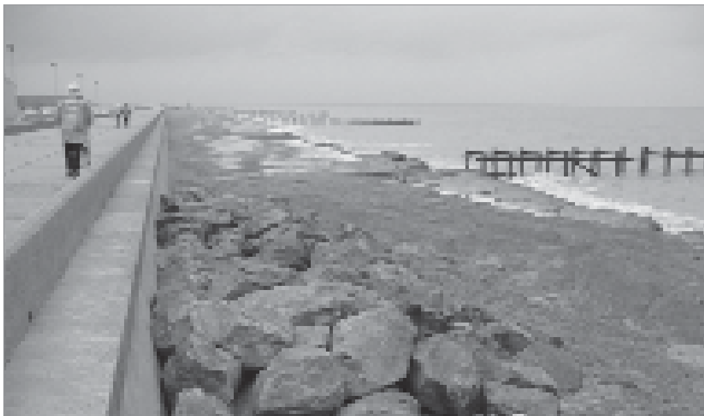
Figure 6.49 Rock revetment to protect a concrete seawall (courtesy Halcrow)
