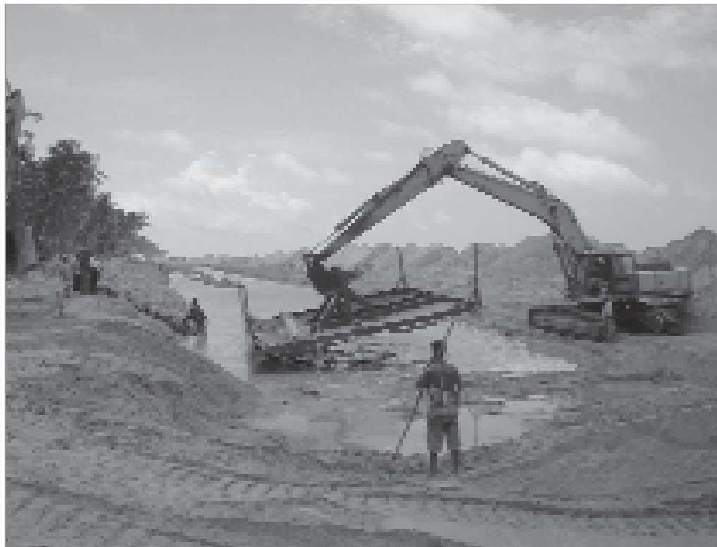
Figure 6.56 Placement of a geotextile using a frame (courtesy HR Wallingford)
