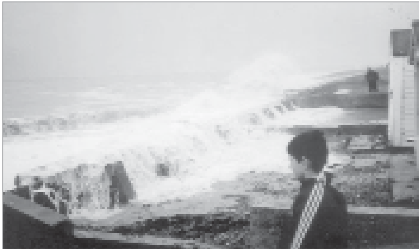
Figure 6.54 Overtopping of seawall. Note pedestrians and proximity of small buildings (courtesy Halcrow)
