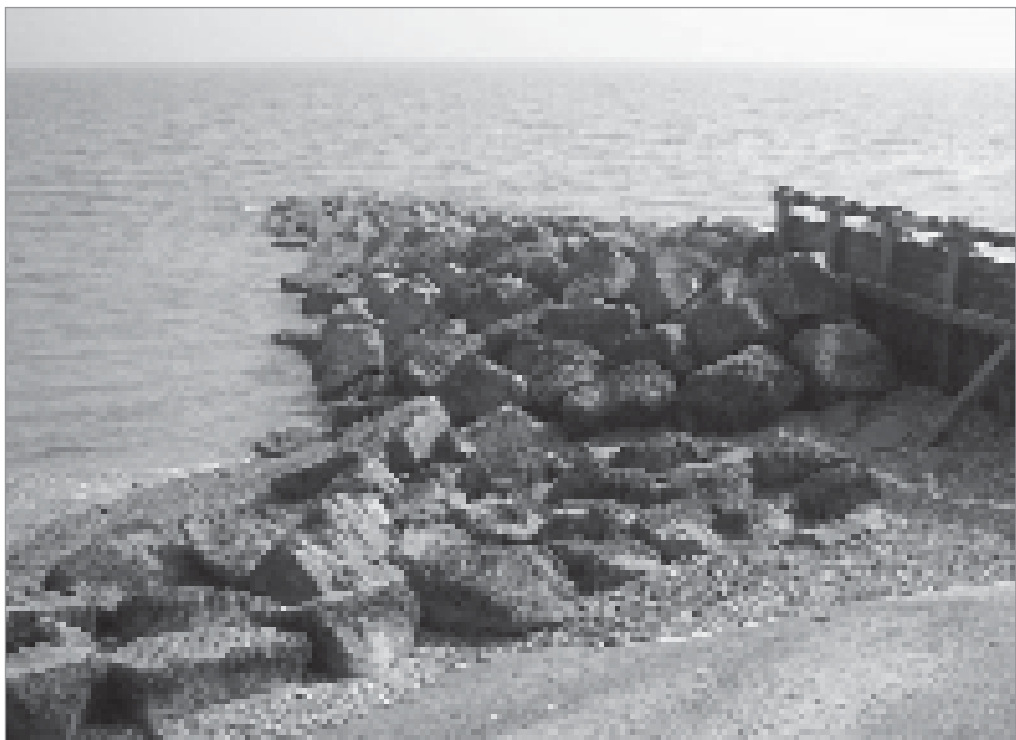
Figure 6.44 Typical rock groyne (courtesy Halcrow)
