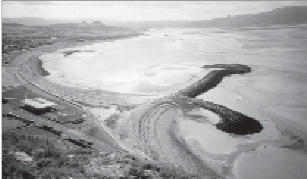
Figure 6.46 Fishtail groyne (courtesy DEFRA/Halcrow)
