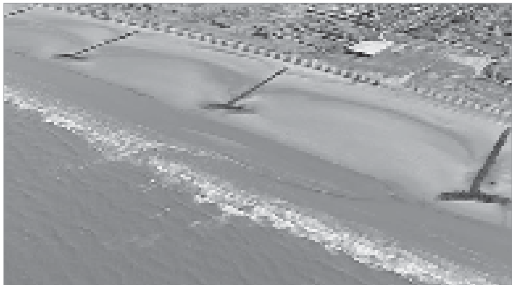
Figure 6.79 T-head groynes, Rhyl, UK (courtesy DEFRA/Halcrow)
