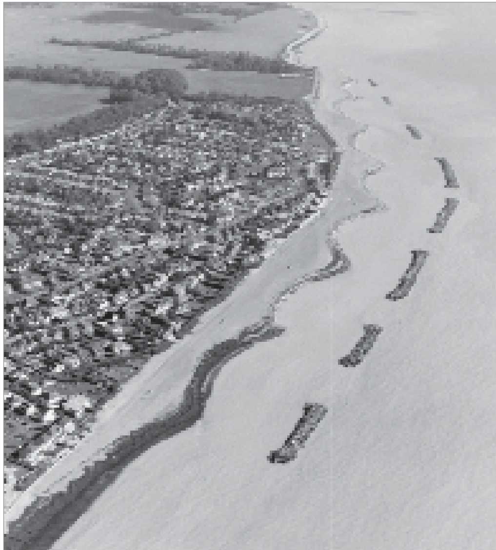
Figure 6.45 Detached breakwaters, Elmer, UK (courtesy Environment Agency/Arun DC)
