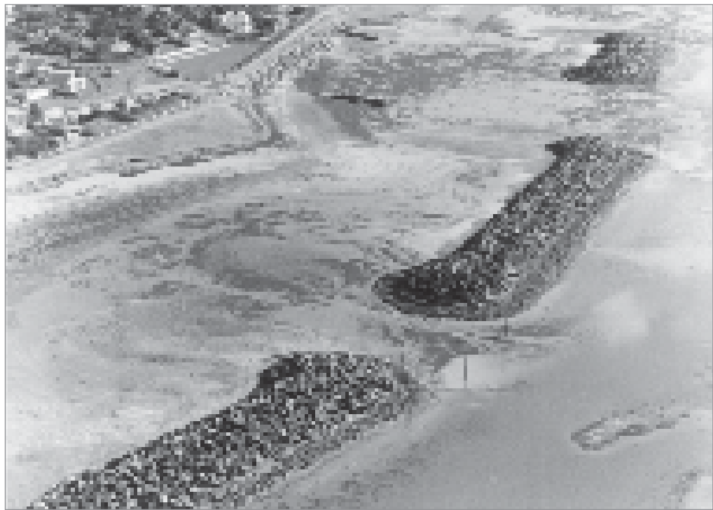
Figure 6.77 Detached breakwaters, Elmer, UK (courtesy Environment Agency)
