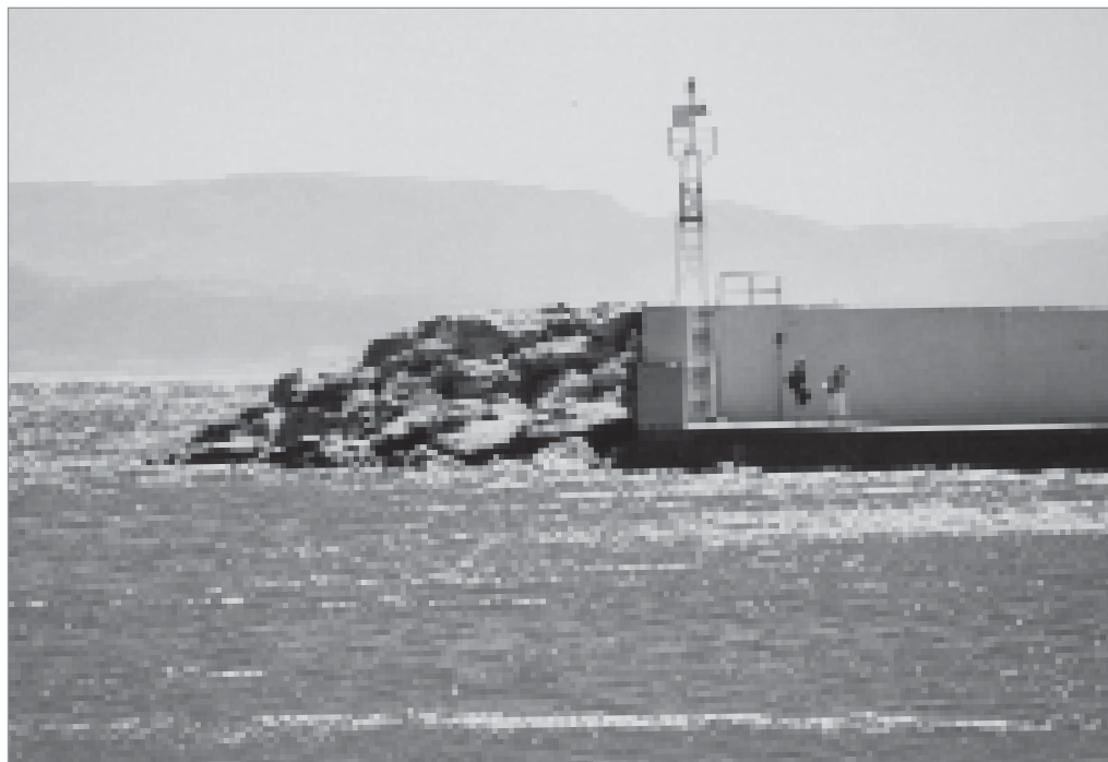
Figure 6.9 Armourstone protection on breakwater roundhead, adjacent to vertical caisson (courtesy Clive Orbell Durrant)
