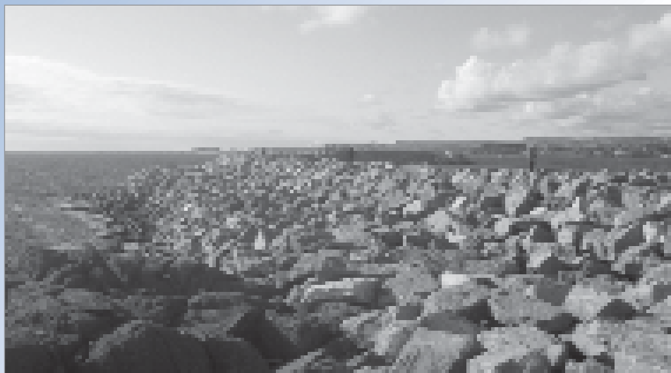
Figure 6.30 View of the front side of Sirevåg breakwater, Norway (courtesy HR Wallingford)
