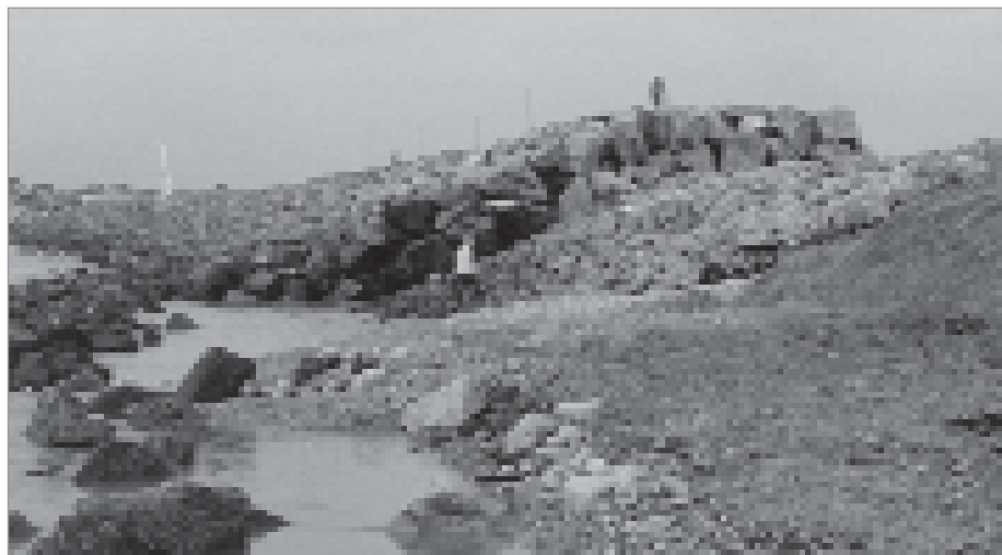
Figure 6.42 Rock revetment, Hurst Spit, UK (courtesy Andrew Bradbury)
