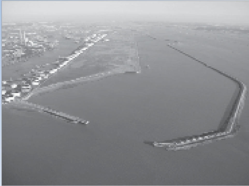
Figure 6.5 Port 2000 Le Havre, France (courtesy Port du Havre)
