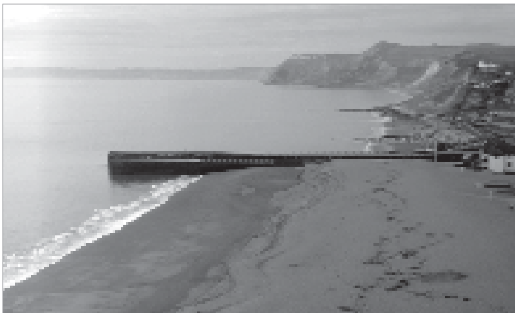
Figure 6.50 Large isolated groyne (harbour arm) trapping sediment (courtesy HR Wallingford)
