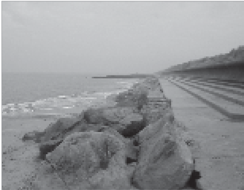
Figure 6.43 Scour protection to seawall, Happisburgh, UK (courtesy Halcrow)
