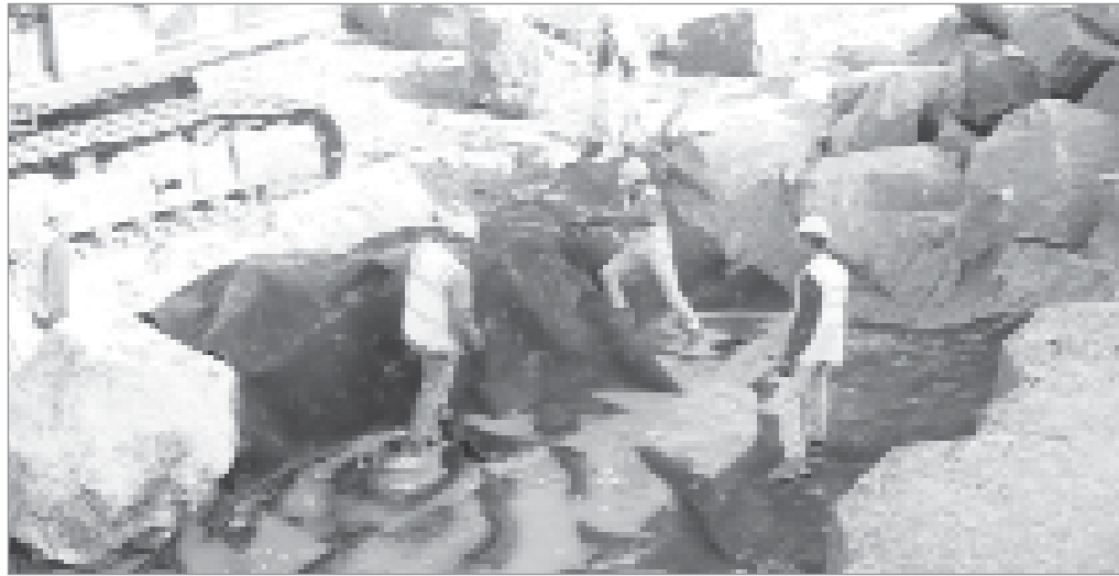
Figure 6.65 Construction of Dutch toe, geotextile being wrapped around toe stones (courtesy Halcrow)
