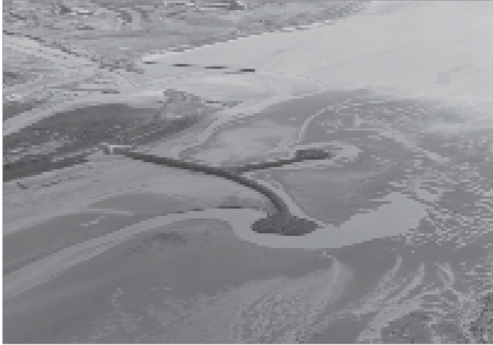
Figure 6.52 Fishtail groyne, Llanelli, UK (courtesy DEFRA/Halcrow)
