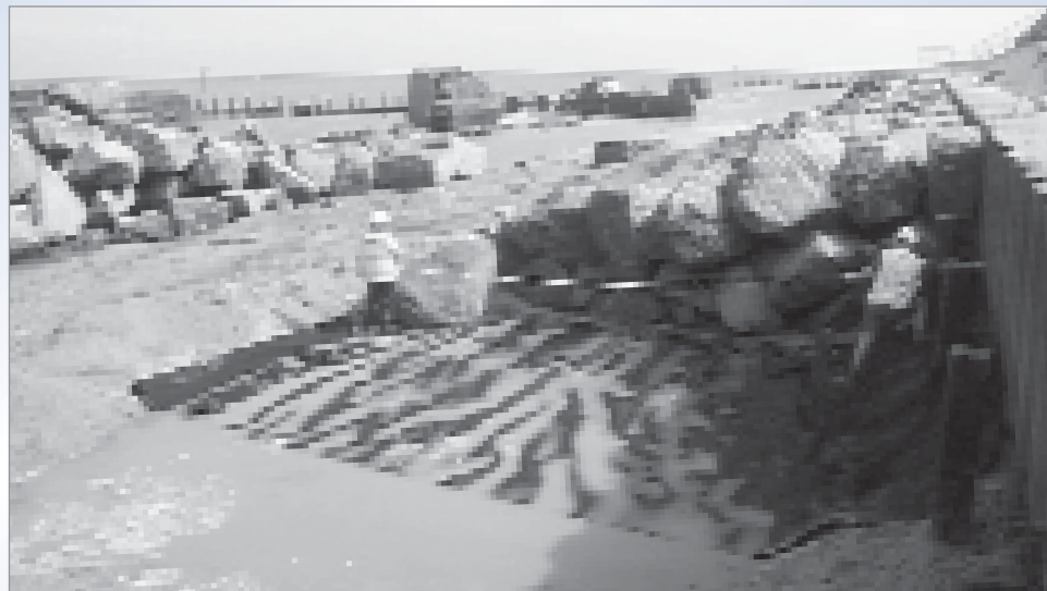
Figure 6.71 Construction of Corton coast protection scheme, UK (courtesy Halcrow)
