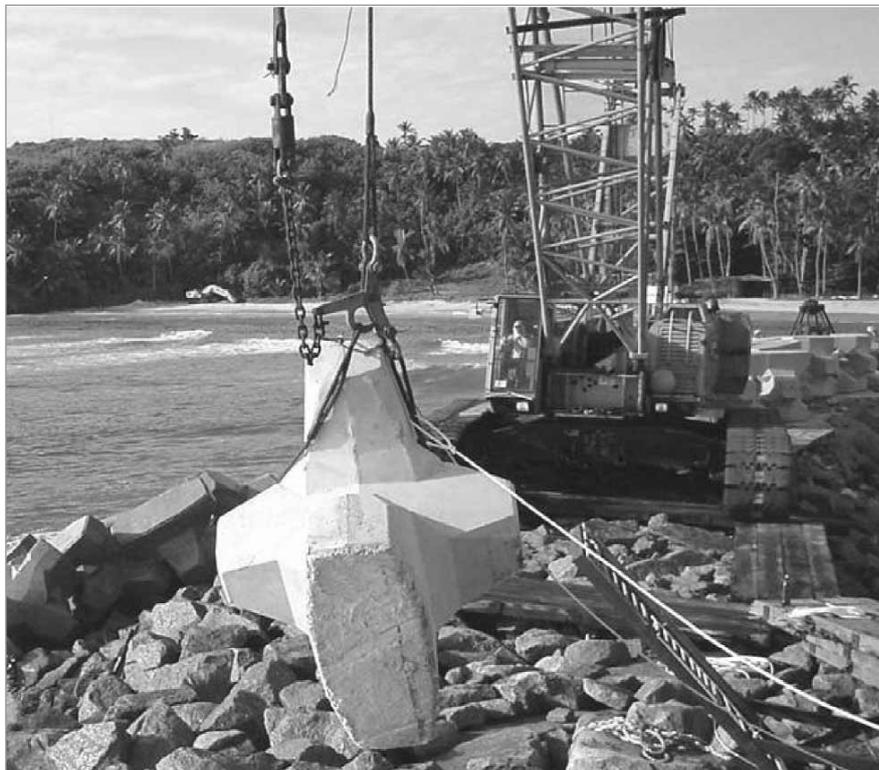
**Figure 9.61** Use of a quick-release hook (courtesy Interbeton)
