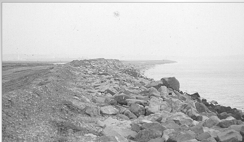
**Figure 10.9** Hurst Spit armourstone revetment in December 1989, after storm damage (courtesy A P Bradbury)
