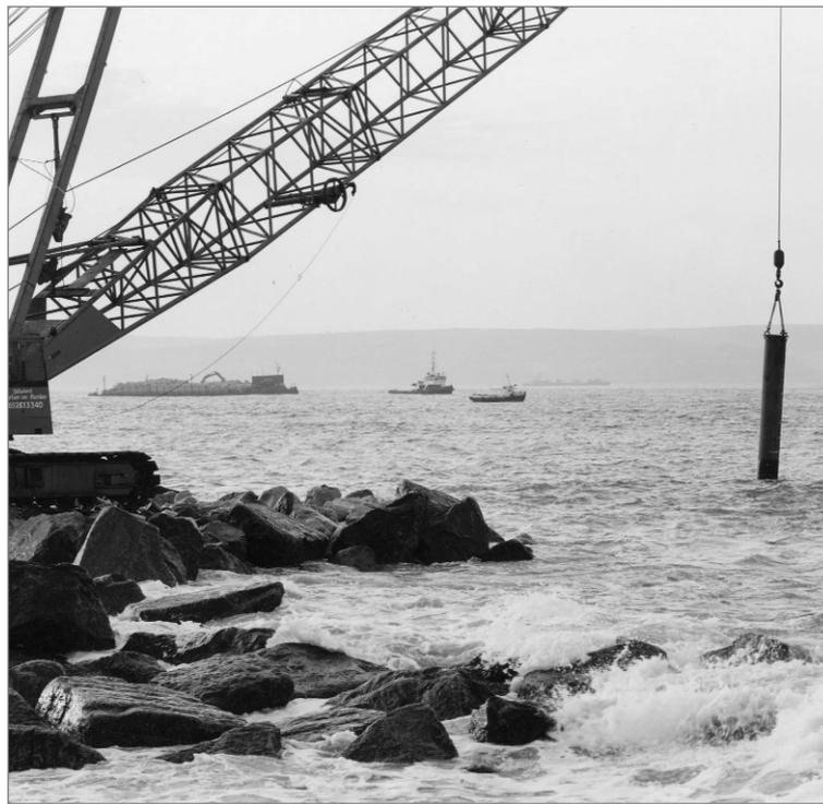
**Figure 10.12** Profiling the submerged section of a breakwater by soundings from a crane (courtesy David Bowie Photographic)
