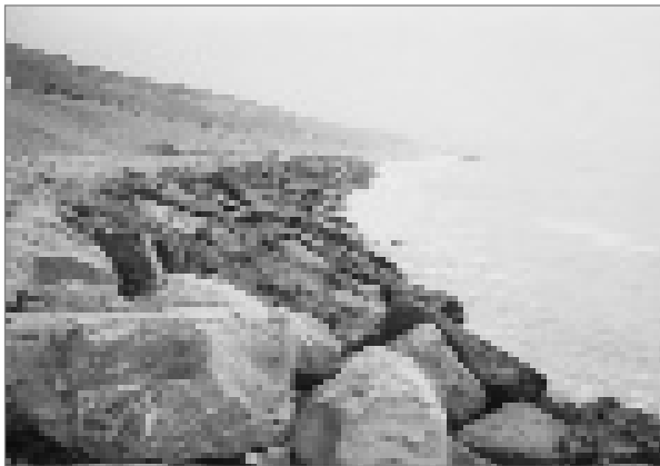
Figure 1.6 Rock revetment (courtesy HR Wallingford)
