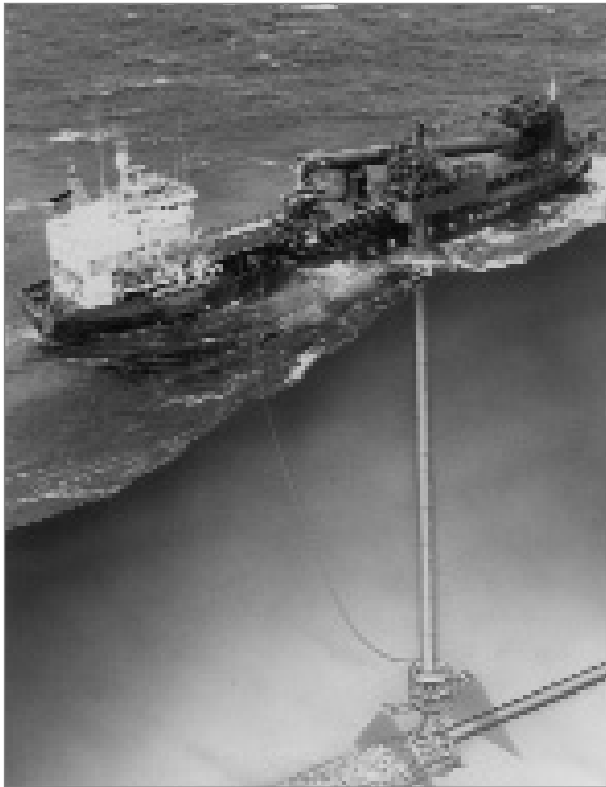
Figure 1.10 Rock protection to pipelines – using a fall-pipe dumping vessel (after CUR 1995, courtesy Van Oord nv)
