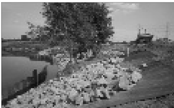
Figure 1.15 Rock revetment being constructed on geotextile (courtesy Mott MacDonald)
