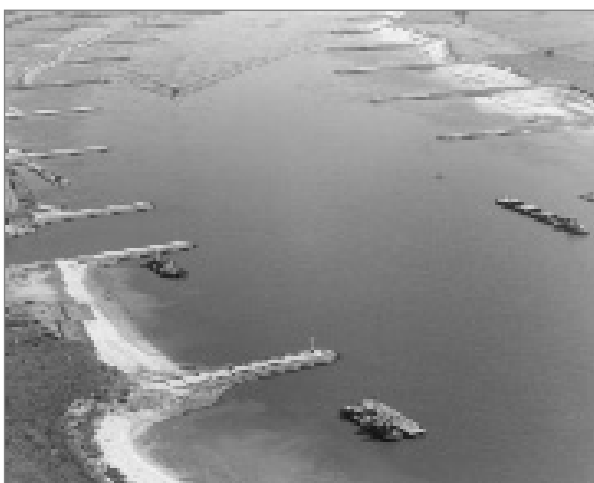
Figure 1.17 Spur-dikes (after CUR 1995)
