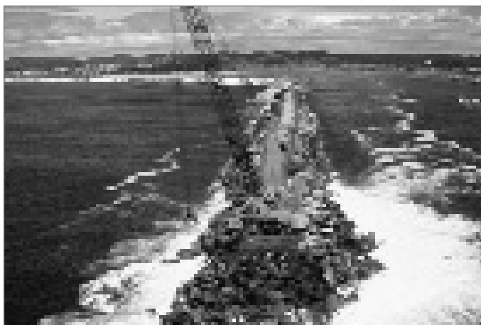
Figure 1.2 Rubble mound breakwater (courtesy Brien Wegner, USACE)
