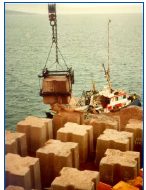
Left: spreading of filter stone; Middle above: scheme of reconstruction of toe; Middle under: Scheme of placement of concrete elements; Right: handling of 65 tons elements.
