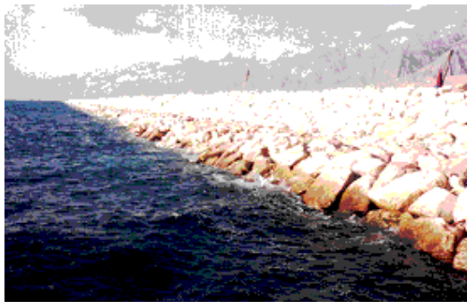
Fig 7: Assaluyeh berm breakwater
