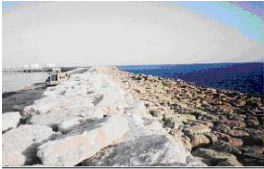
Fig 9: Chabahar berm breakwater
