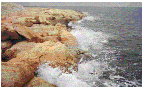
Fig 15 : Damage of edge in Berm
