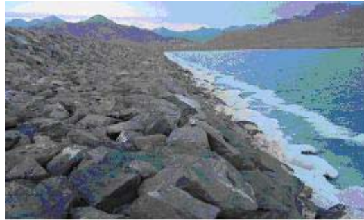
Fig 10: Urmia berm breakwater
