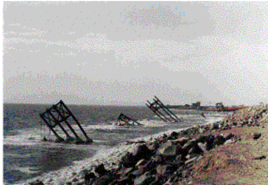
Fig 19: Squeezing out the subsoil , Urmia
