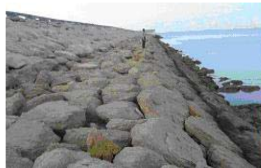
Fig 8: Basaedu berm breakwater
