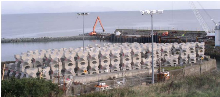
Figure 7: Storage of Xbloc armour units
