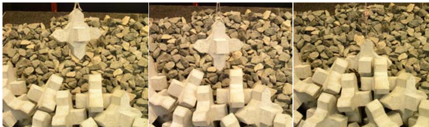
Figure 9: Xbloc placement pattern (placement of scale units)
