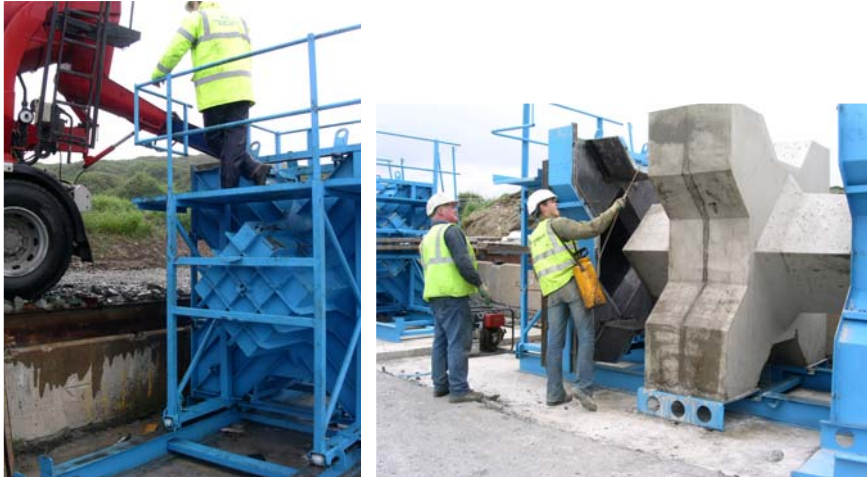
Figure 6: casting and curing of Xbloc armour units
