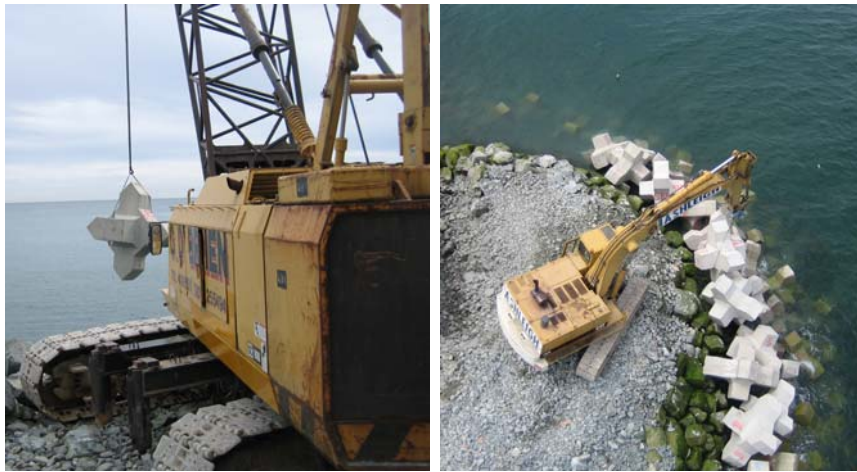
Figure 10: Xbloc placement a) by crawler crane and b) by excavator
