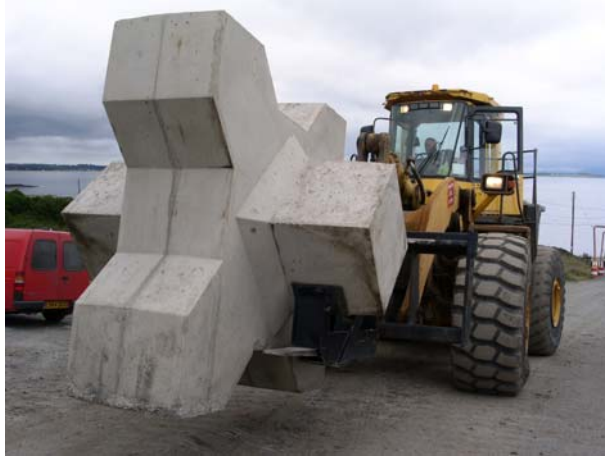
Figure 8: Handling of Xbloc armour units
