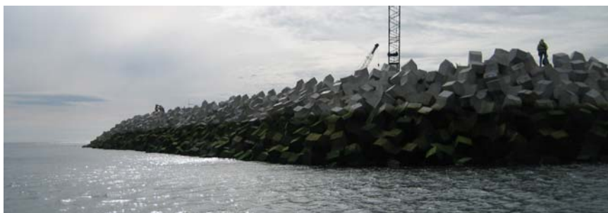
Figure 11: Impression of breakwater slope covered with Xblocs
