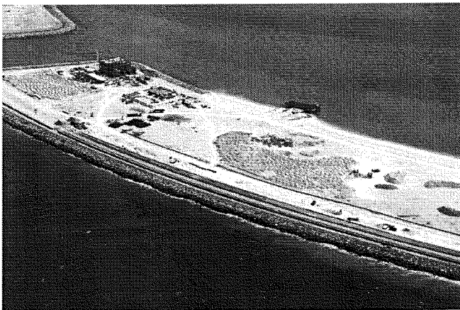
Palm Jumeirah, outer face of crescent breakwater
