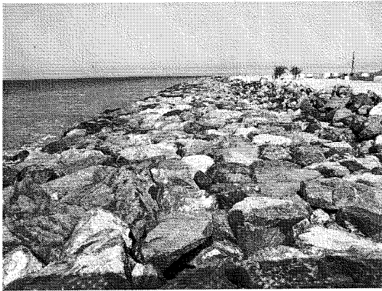
Crescent breakwater 20 m rock crest width
