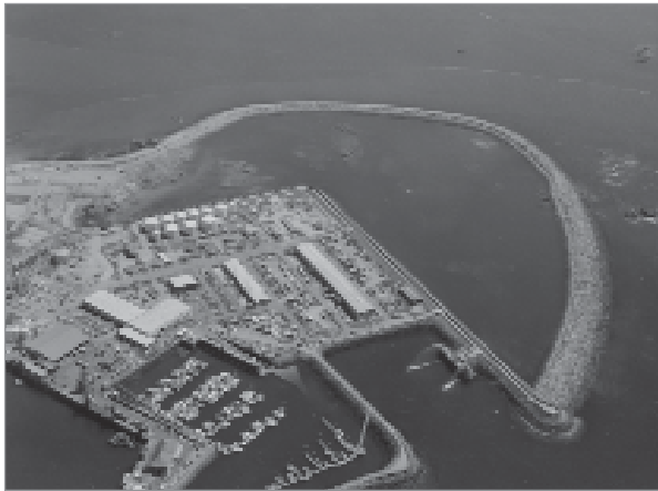
Figure 1.4 Breakwater – eventually to contain reclamation (courtesy Edmund Nuttall)
