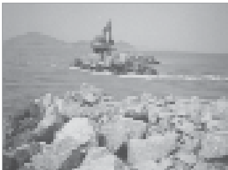
Figure 1.11 Rockfill closure dam under construction (courtesy KARICO)
