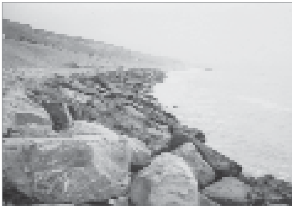
Figure 1.6 Rock revetment (courtesy HR Wallingford)
