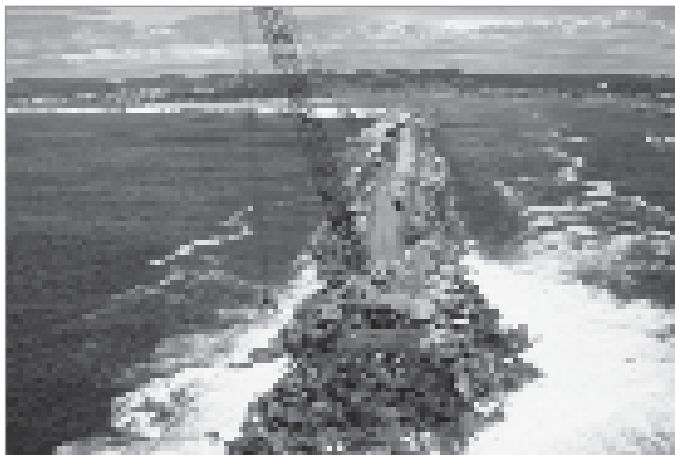
Figure 1.2 Rubble mound breakwater (courtesy Brien Wegner, USACE)
