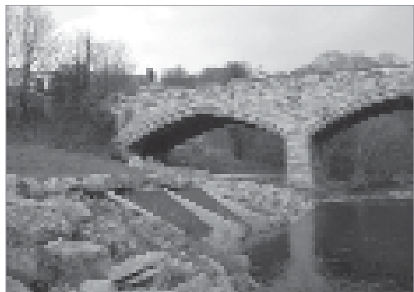
Figure 1.16 Rock protection to outfall structure on bank (courtesy Charlie Rickard)
