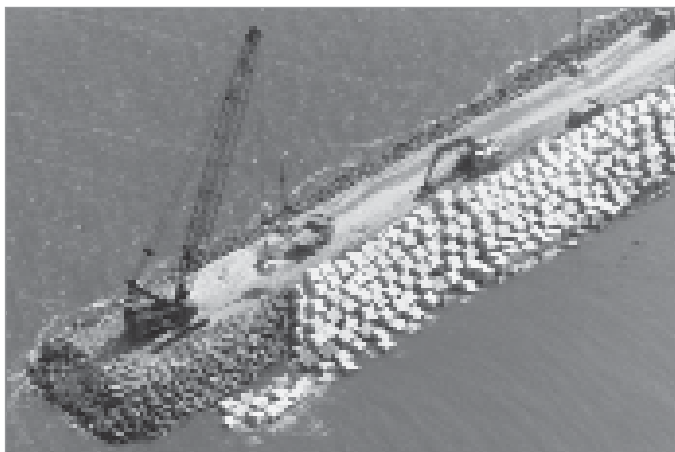
Figure 1.3 Construction of breakwater using concrete armour units (courtesy CUR)
