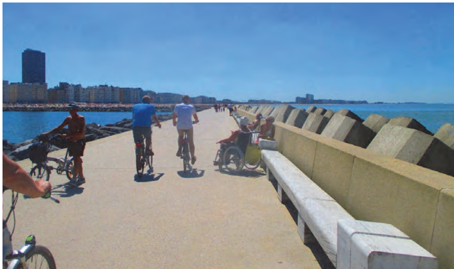
Figure 3.16 New breakwater at Oostende, Belgium, with a main function of access for people
