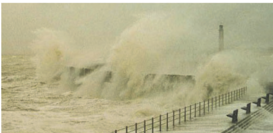
Figure 3.2: Spray overtopping at the breakwater at Margate, UK
