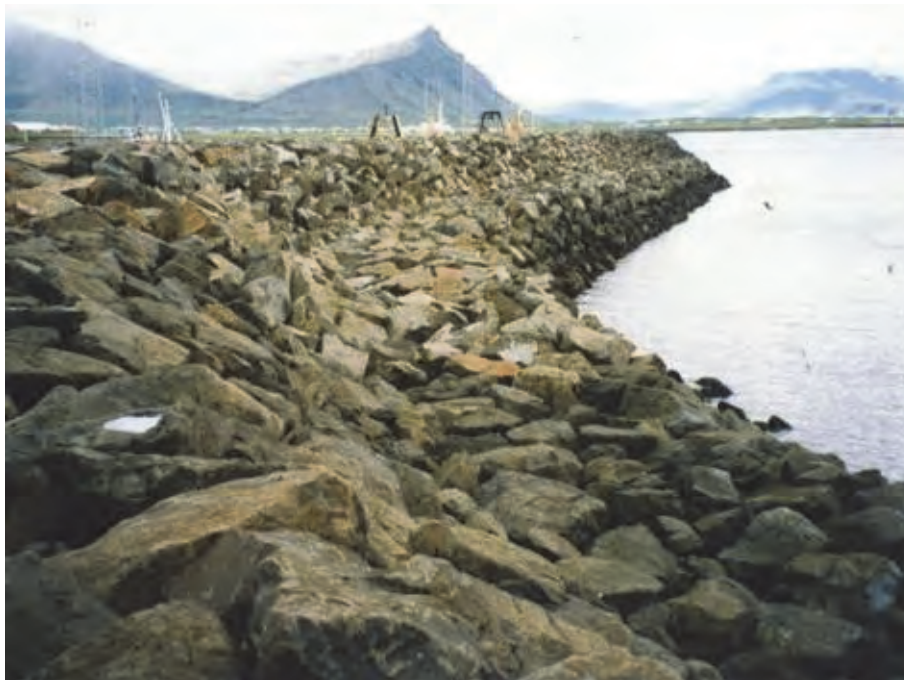
Figure 6.10 Icelandic-type berm breakwater
