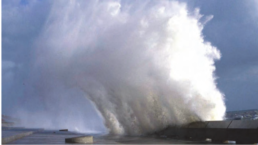
Figure 3.17 Severe wave overtopping at Samphire Hoe, UK.
