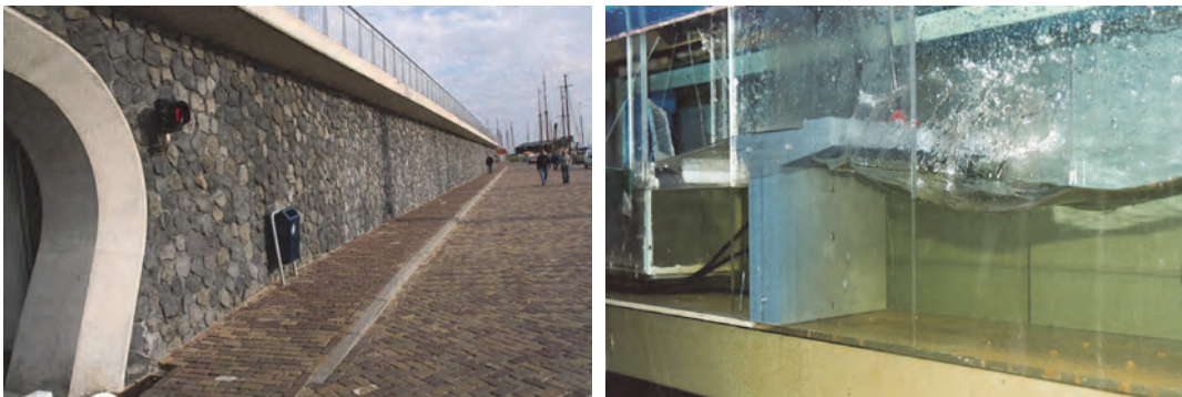
Figure 1.9: Large and effective wave return wall at Harlingen (NL). The wave return wall is part of a promenade on top of the wall (picture above). Lower left: the wall with wave return wall in reality; lower right: model testing under design wave conditions
