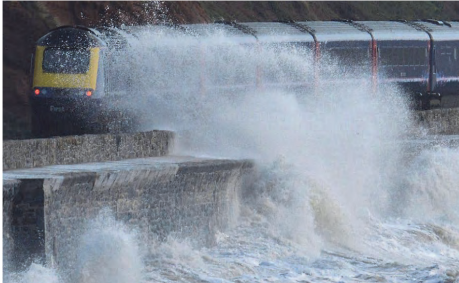
Figure 3.23: Wave overtopping onto a moving train, UK
