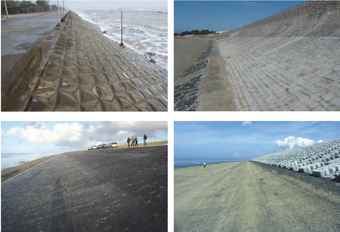
Figure 5.2: Examples of coastal dikes, levees and seawalls. Hanoi, Vietnam; Ile de Ré, FR; Boonweg, NL; Hondsbossche zeevering, NL
