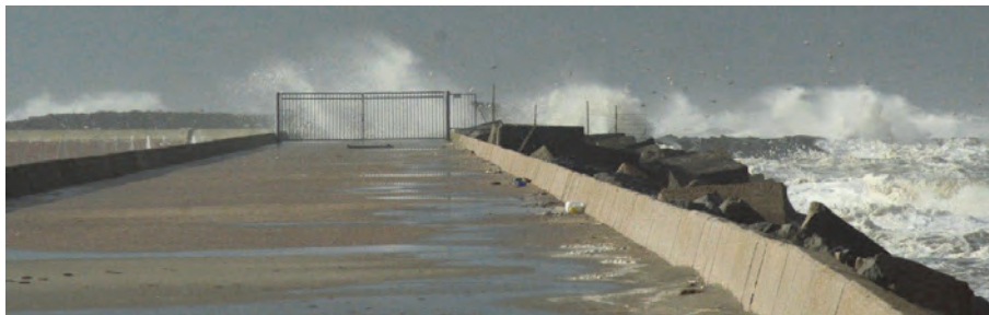
Figure 3.15 Severe wave overtopping and wave transmission at the breakwater of IJmuiden, the Netherlands
