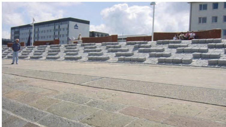
Figure 5.26: Example of battens or ribs in reality
